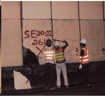
路政署須拆卸承判商未有更換的石棉板塊 Highways Department takes remedial action to remove asbestos panels which a contractor failed to replace
