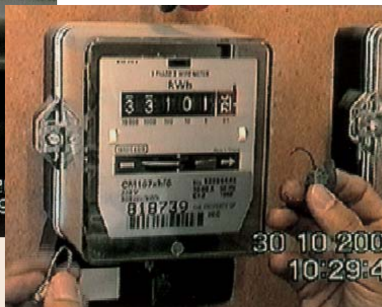
經仔細檢查後發現電錶被干擾 Meter tampering revealed on close examination
