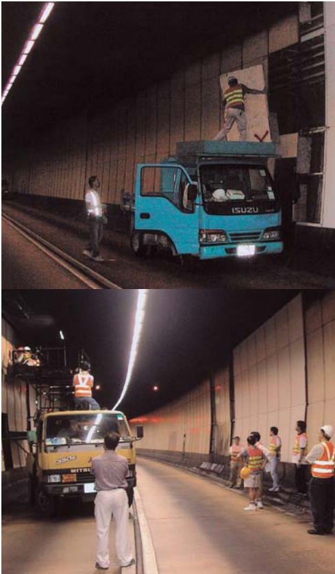
路政署須拆卸承判商未有更換的石棉板塊 Highways Department takes remedial action to remove asbestos panels which a contractor failed to replace
